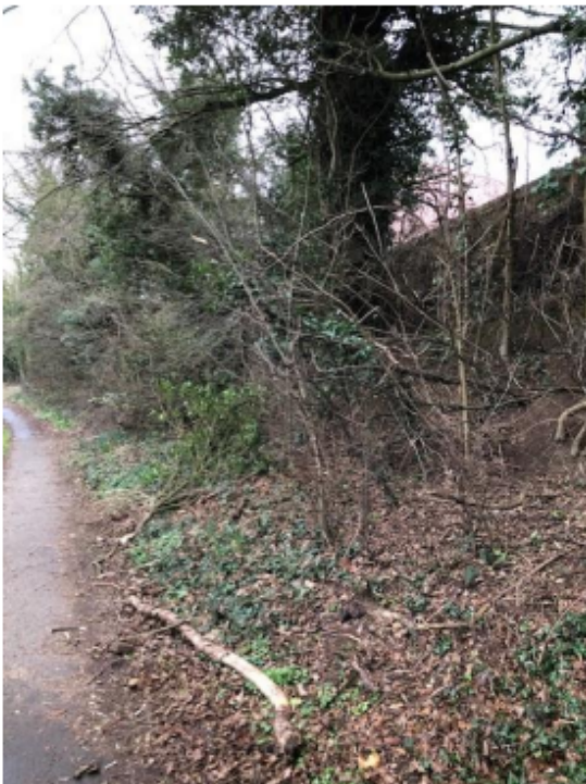
Figure 2: The Cambridge Road verge requiring much TLC before FP3 is installed.
