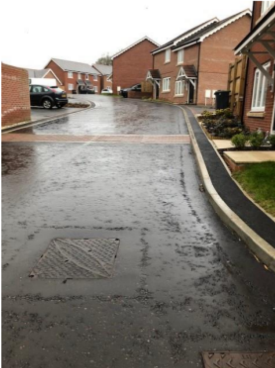
Figure 1: The steep incline of King Charles' Drive looking towards the affordable homes and showing the sub-standard width of the footway.
